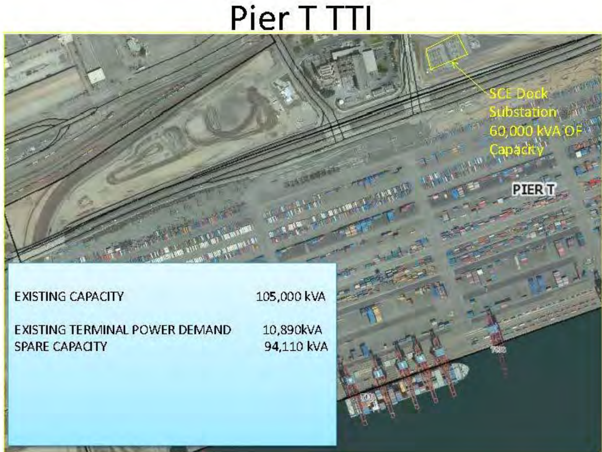
Figure 6: Pier T TTI– Electrical Capacity and Demand
